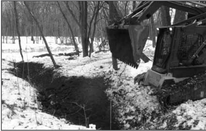
Soil block installation at Salt Creek Nature Preserve.
