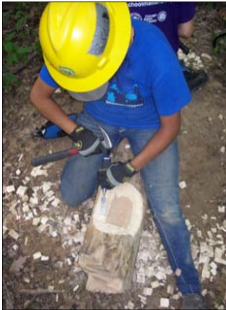
Left: An intern takes the bark off a log to use it as a check step for erosion control on a trail at Dan Ryan Woods; Right: High school interns Ida Harden, Giovanni Gonzalez, Gloria Orozco and Yasmine Khazneh.
